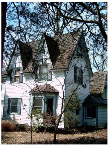
Roof planes broken via multiple dormers.
