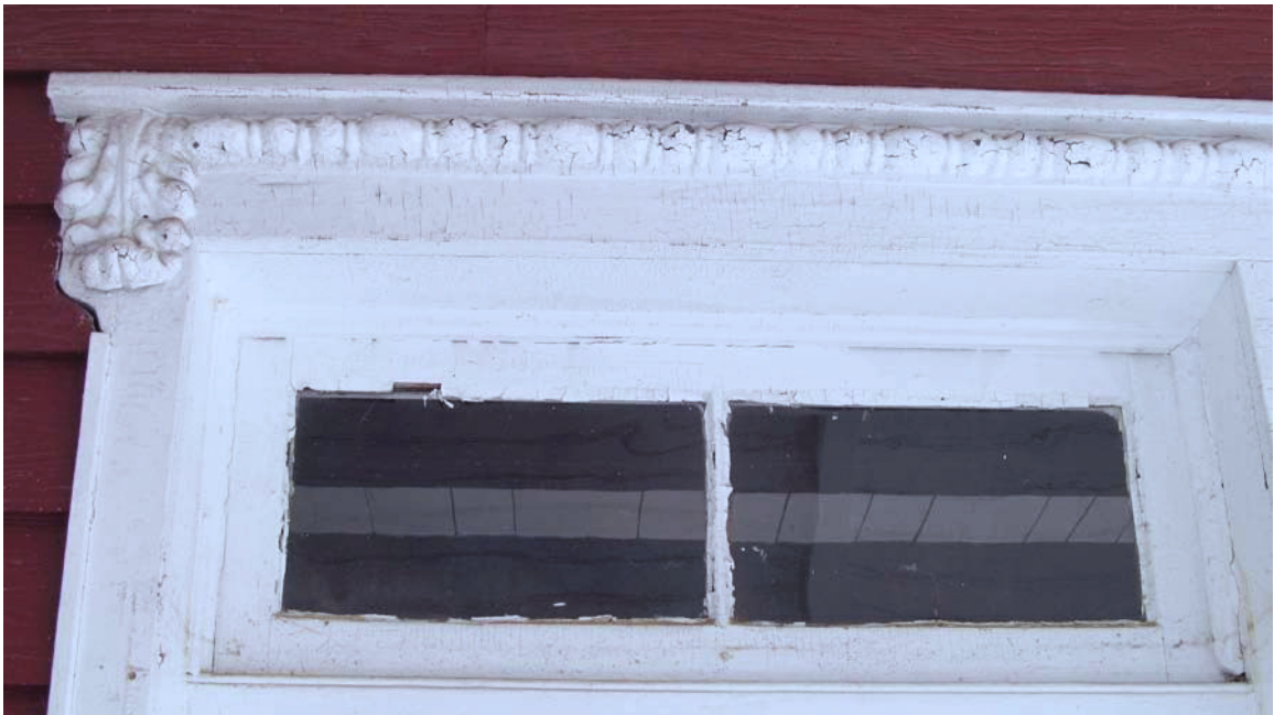
Figure 4a (315 Grove Avenue) Detail of Original House Façade Under Porch Roof Original Transom Window with Applied Decoration
