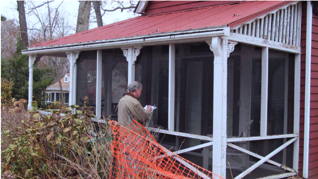
Figure 3 (315 Grove Avenue) East Elevation of Second Avenue Porch Showing Square Posts, Vertical Board Lattice Zigzag Rake Board & Sawn Board Brackets
