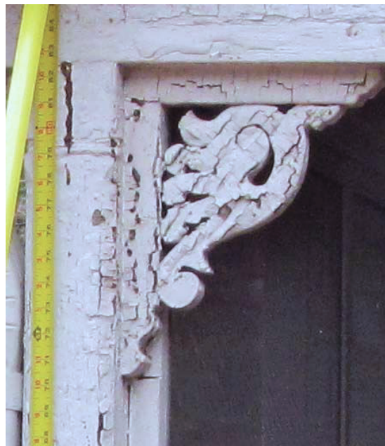
Figure 3a (315 Grove Avenue) Second Avenue Porch Details Sawn Board Bracket, Square Post with Chamfered & Incised Details
