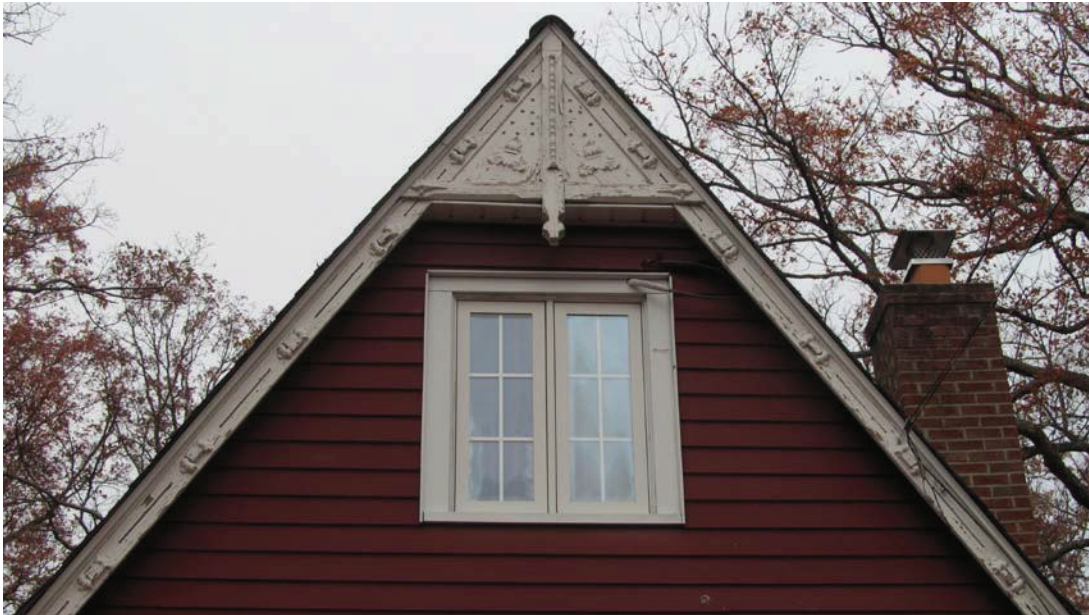
Figure 5 (315 Grove Avenue) Original House Façade Above Porch Roof, Deep Main Roof Overhang Barge Board & Flat Board Pediment
