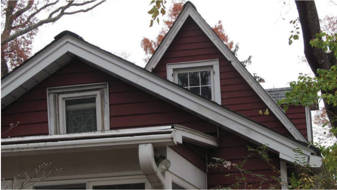
Figure 6 (315 Grove Avenue) Rear Elevation (Detail) Shallow Gable Addition and Roof Overhang
