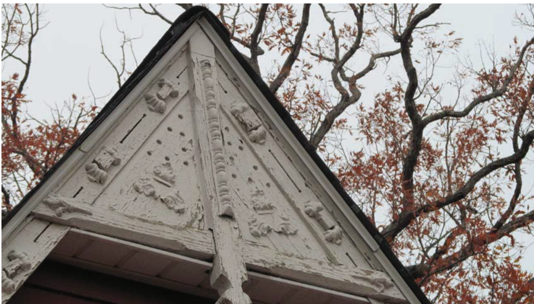
Figure 5a (315 Grove Avenue) Barge Board Details: Applied Acanthus Leaves & Blocks Flat Board Pediment Details: Paneled Soffit, Drilled & Applied Decoration, Drop Finial
