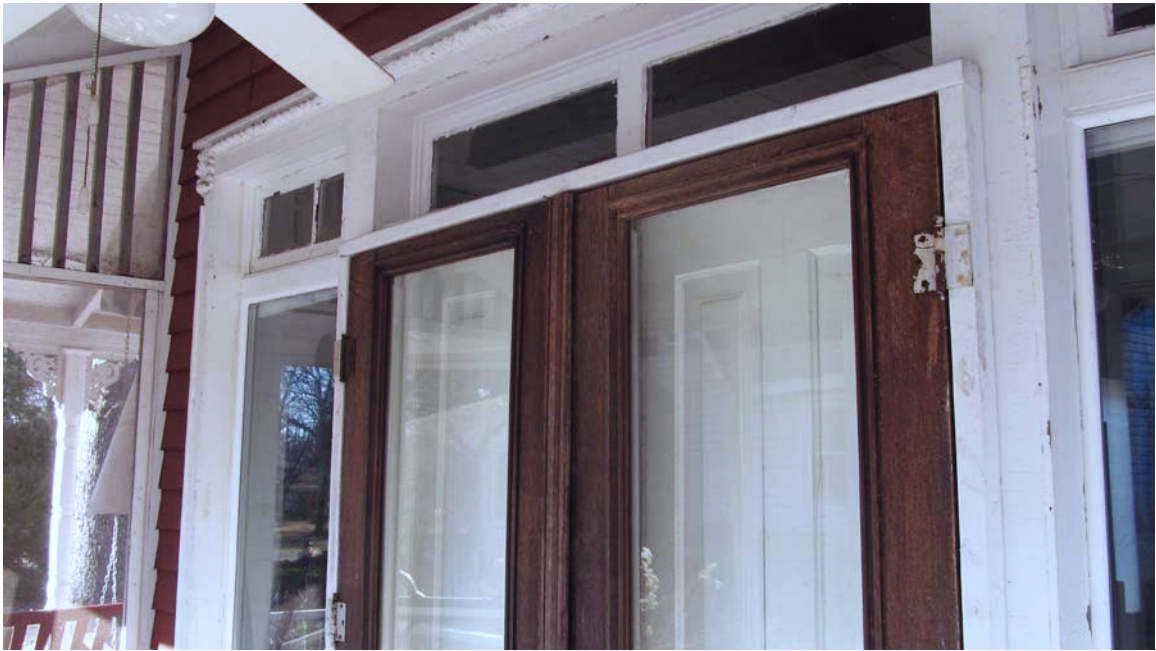
Figure 4 (315 Grove Avenue) Original House Façade Under Porch Roof Original Door and Window Casings, Original Transom Windows, Lattice Triangle
