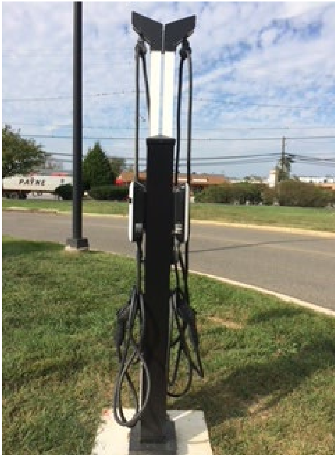
Peppo Level 2 design for a pair of chargers (Note the 3' x 3' pad and bollards are not shown)
