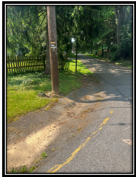
Figure 2. Asphalt swales need to be replaced with bio swales to treat water before it hits storm drain and reaches West Woods.
