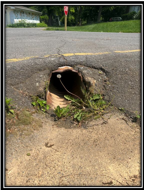
Figure 1. Undersized CMP.
