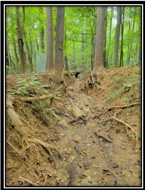
Figure 9. Channel with minimal hindrance to erosion and severe entrenchment causing all flood flows to be contained in the channel and increase pressure on the banks.
