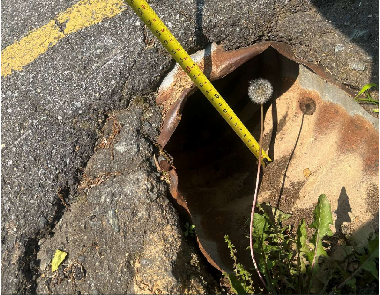
14" SD at invert in Southeast Corner of Hickory Road and Center Street Intersection
