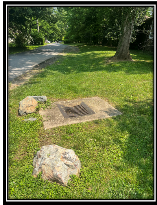
Figure 3. Varying types of structures onsite could be replaced with more efficient structures that can handle a larger capacity and further prevent overland flow from bypassing structure and creating runoff in west woods.
