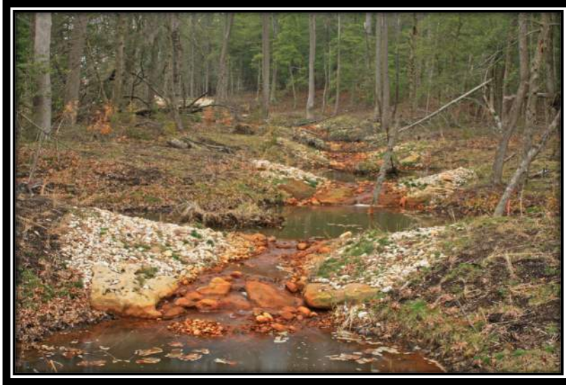
Figure 26. Regenerative Step Pool Storm Conveyance Example.
