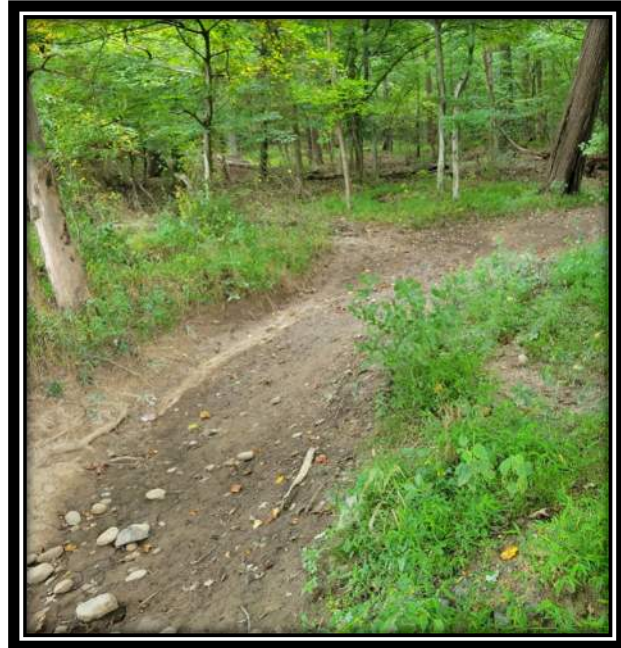
Figure 16. Area where pipe was removed and "ford" was by default created. Backwater is causing washout of the upstream portion.
