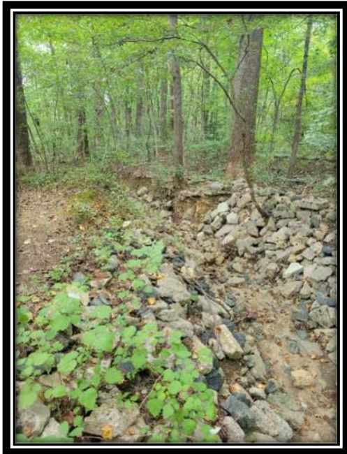
Figure 13. Looking downstream of the Culvert. Trees are compromised right at the downstream limits of rip-rap armoring.
